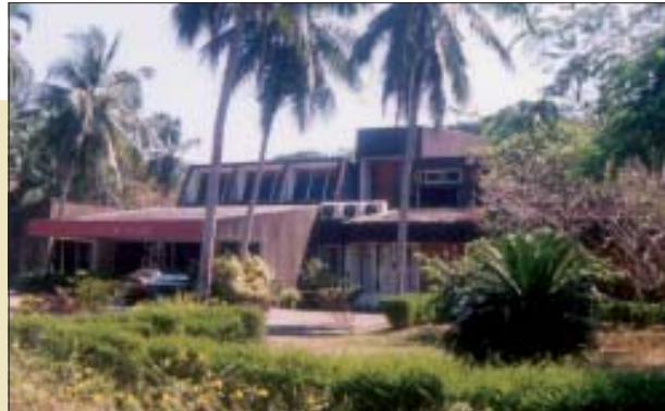
Chitranjali Studio, Thiruvallam – the indoor studio is one of the biggest in the country, in terms of floor area.
