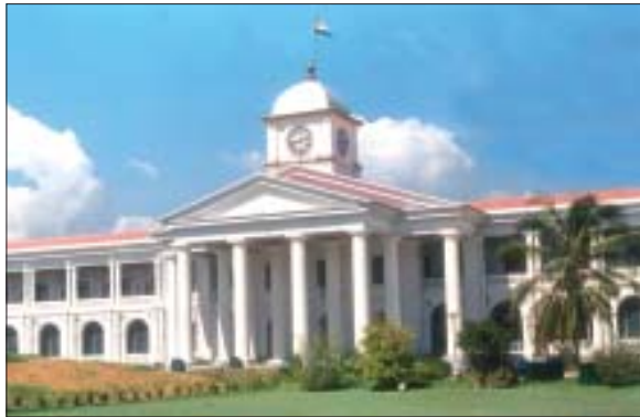
The Kerala Government Secretariat building – the seat of the State administration. This imposing building in the lines of Roman-Dutch architecture, was built during the reign of H.H. Ayilyam Thirunal Rama Varma, Maharaja of Travancore who reigned from 1860 to 1880.
