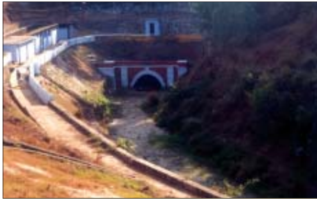
The defunct water way tunnel at Varkala
